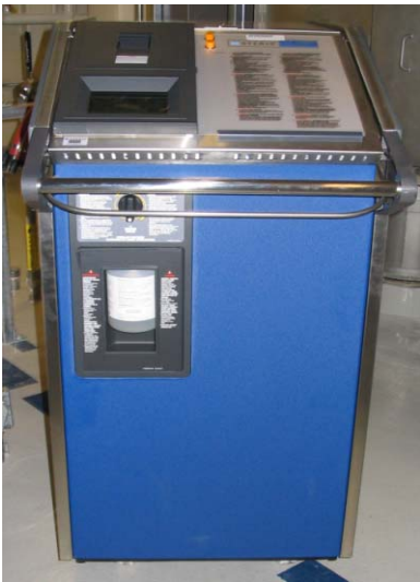
Fig. 2: Front view of the VHP generator (STERIS® VHP 1000ED) located on the penthouse mechanical space. VHP was piped into the lab for the biodecontamination process
